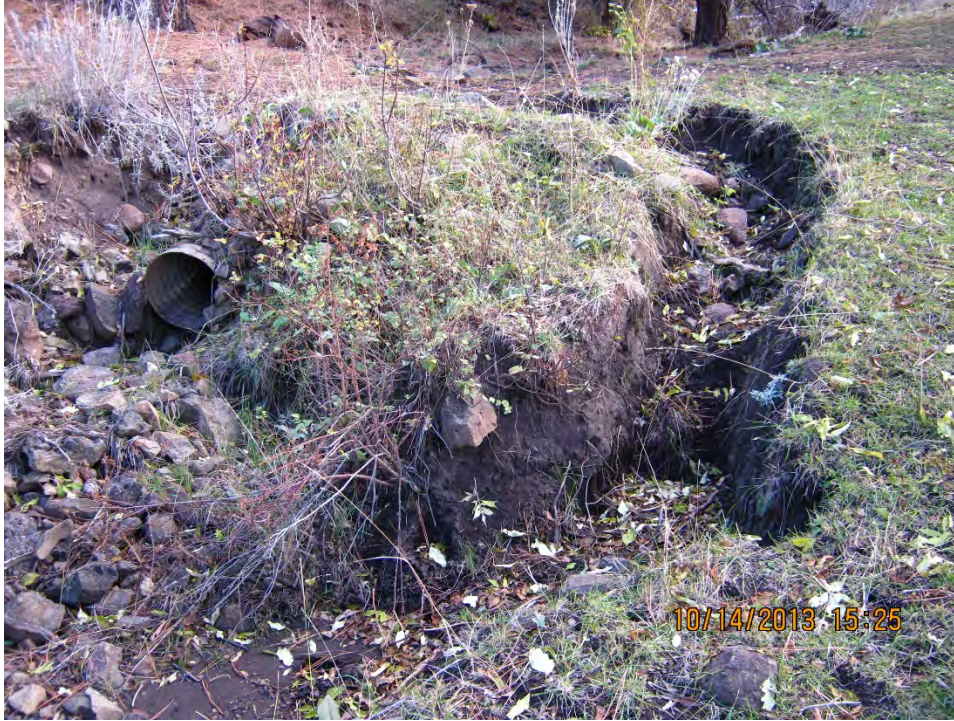
UN_G_127. View to north. Stream has eroded a channel across the road instead of going through the culvert.
